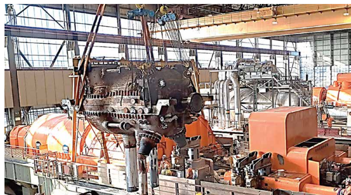
Figure 7. Unit 3 IP turbine section being moved to replace the Unit 2 IP section.
