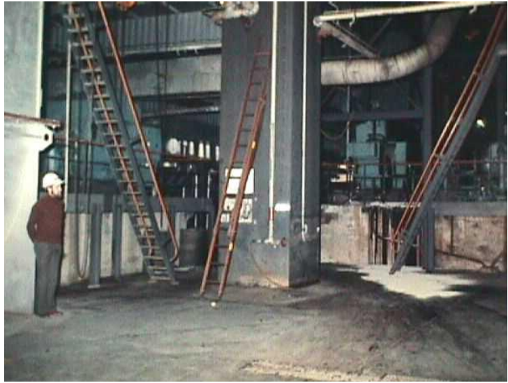
Figure II: main corner column and the two adjacent mills.
