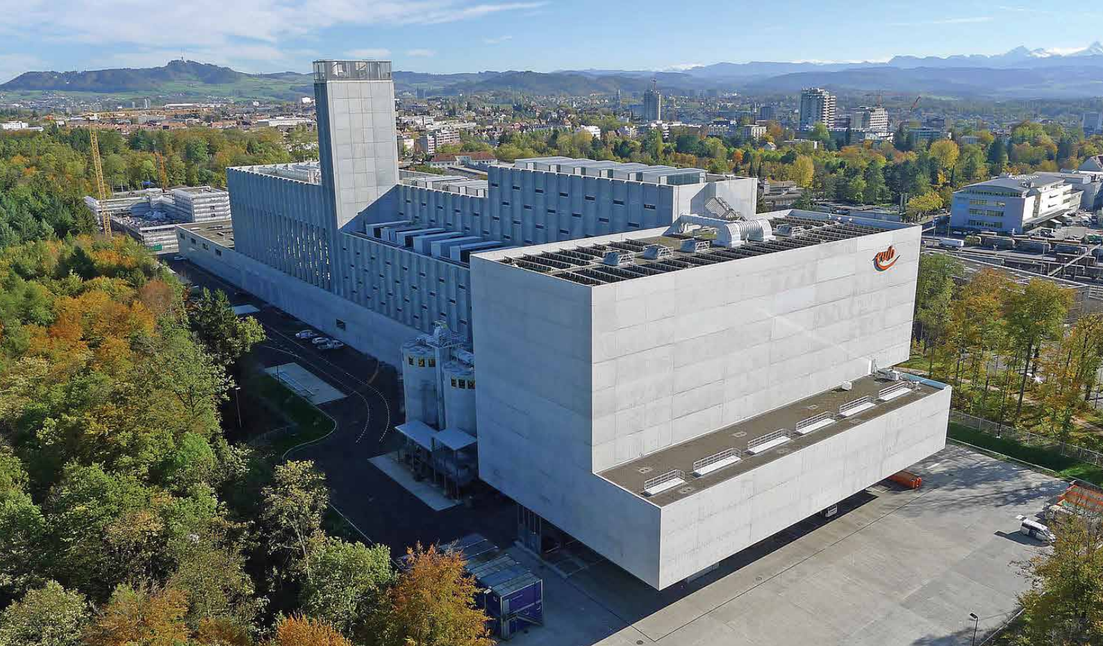
Figure 1: Energiezentrale Forsthaus in Berne, Switzerland.
