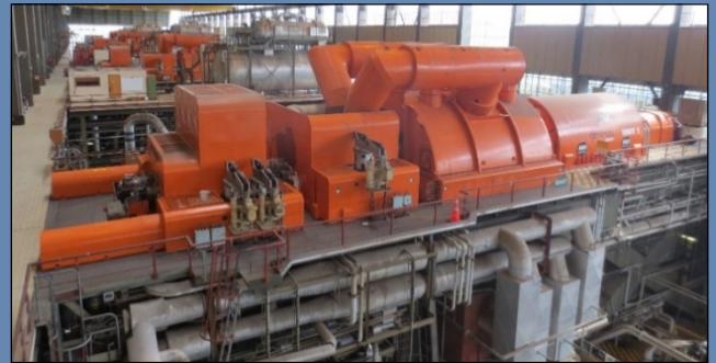
Figure 2. Rankine Unit 1. Rankine refers to the thermodynamic cycle of the steam turbines, which are Units 1 to 4. Other generating units at Huntly include Unit 5, which is a 385 MW combined cycle plant (Rankine and Brayton cycle) and Unit 6, which is a 50 MW gas turbine for peaking (Brayton open-cycle).
