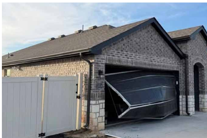
Above: Deflagration risk becomes critical when vent gases accumulate in enclosed or semi-enclosed spaces. Below: * Safety refers to how resistant the chemistry is naturally to entering an uncontrolled state or thermal runaway. Rankings are comparative and do not replace cell, module, pack, charger, installation, or duty-cycle risk assessment. Bottom right: In enclosed spaces, gas accumulation and delayed ignition can dominate the risk profile.
