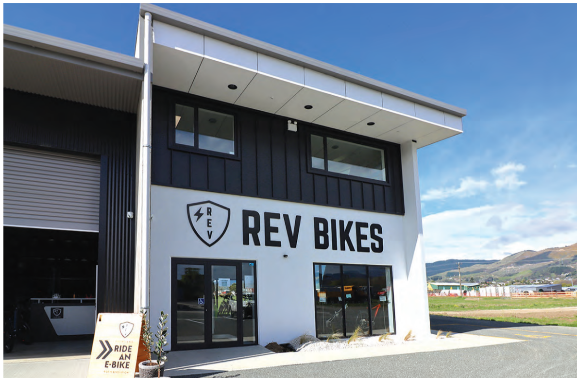
Rev Bike Richmond located at 28 Appleby Highway includes a permanent workshop and showroom. Based just a few metres from the Great Taste Trail, it is the perfect location for customers to take a bike for a test run.
