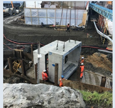
Sections of the new culvert during construction
