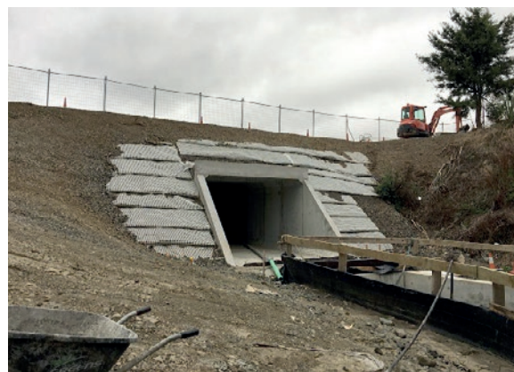
Newly installed culvert, upstream end
