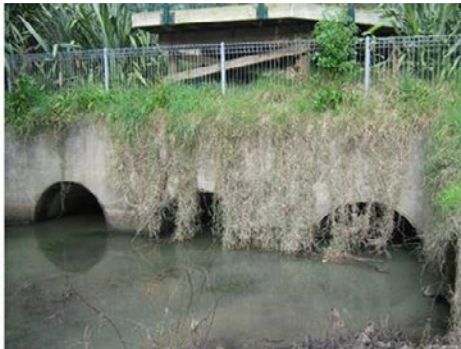
Culvert 2: Waitahurangi stream.
